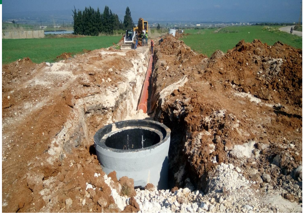
Excavation, pipe laying and manholes construction along primary line MC (January 2016)
